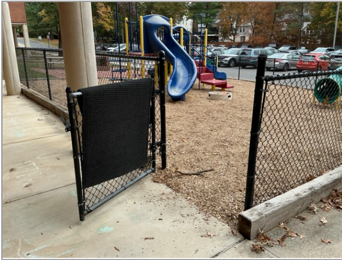
ACCESSIBLE ROUTE TO PLAYGROUND
