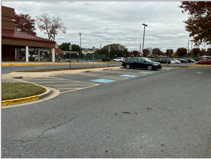
OVERVIEW OF ACCESSIBLE PARKING AREA
